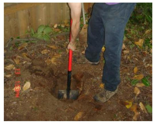
We were hitting roots near the surface so we used a root-hacker tool I had made from a 4 inch cold chisel welded to a piece of 3/4 inch water pipe.
