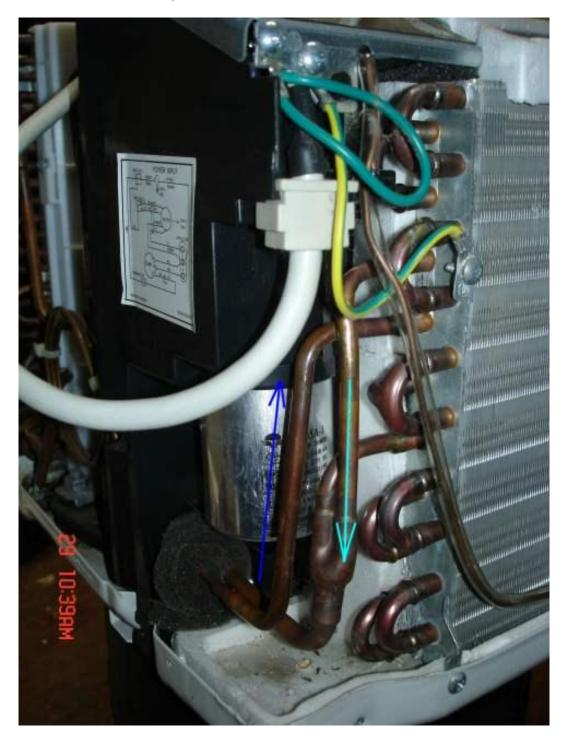
Here's another detail of the tubing near the condenser:
