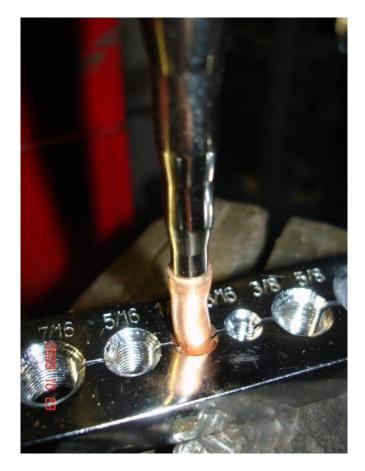
Here I'm using the flaring tool as a vice and I'm tapping the tubing expander with a hammer to stretch the tube to the right size. I'm actually going two steps bigger, so the tubing got a bit deformed, but it ends up being a sound joint.
