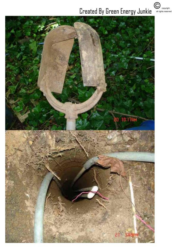
this shows the hole I'm doing the tests in. I used CPCV pipe (not recommended) with a double-loop (not much advantage over a single loop)...
