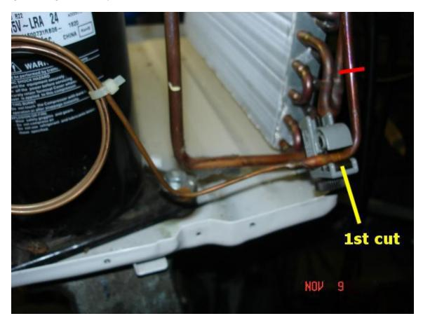
I have made a red mark on the photo to indicate another good place where the cut could have been made...
