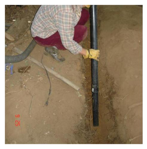
As I stated previously, I though I'd need to use barbed connecctors in the trenches, but later realized that I could pull the pipe up tight, weld the connection, working just inside the trench and then push the pipe in and cover it while holding it down with anything heavy (like large stones or my foot).
