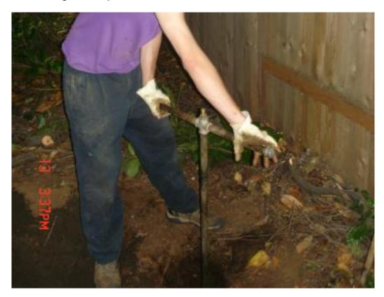
So we warmed up the heater, fused some pipe lengths onto the U-Turn, waited a bit for things to cool off, then down the hole with the poly pipe:
