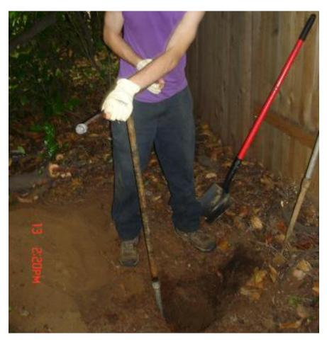
...soon we were down to the end of the extention. We also determined that a bit of water helped the mostly sand adhere better, and made it stay on the auger head while we lifted it to the surface"
