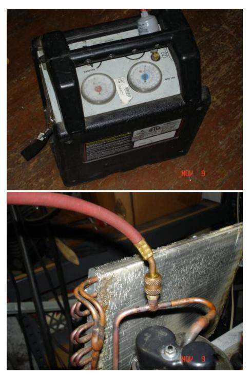
The bottom photo shows the vacuum hose connecting to the previously brazed Schrader valve on the AC unit.
