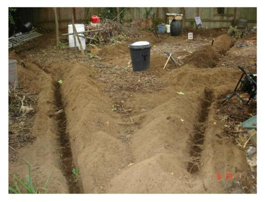
I found that it really pays to run the trencher as close as possible to the plastic pipe, without hitting the plastic. Making corrections for a wide space (I had many) has been very time consuming.
